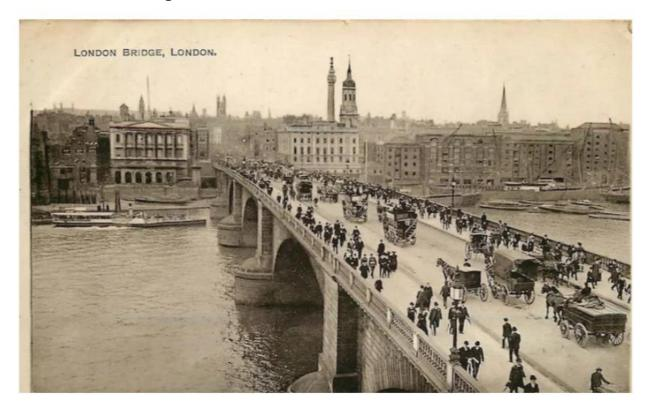
By the end of the 18th century, the London Bridge needed to be replaced. It had fallen into severe disrepair and was blocking river traffic. The "New" London Bridge was completed in 1831, designed in 1799 by Scottish engineer John Rennie. Due to the weight of automobile traffic crossing the bridge in the early 20th Century, it began sinking into the River Thames. By 1924, the east side of the bridge was some three to four inches lower than the west side.
